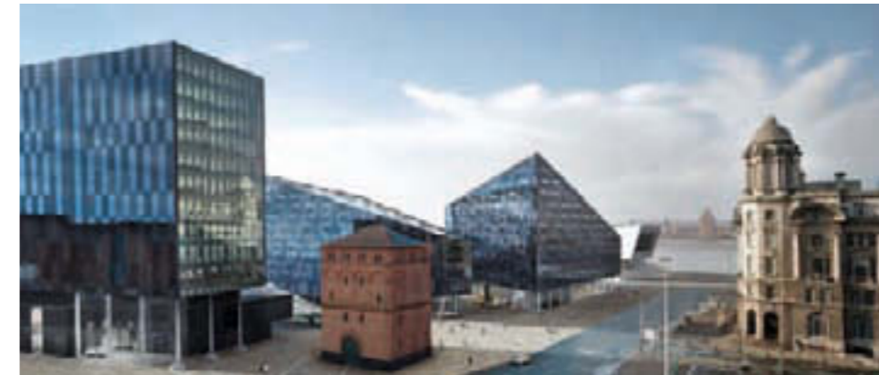
State-of-the-art architecture in a port laden with history – Block 3 on Mann Island.
