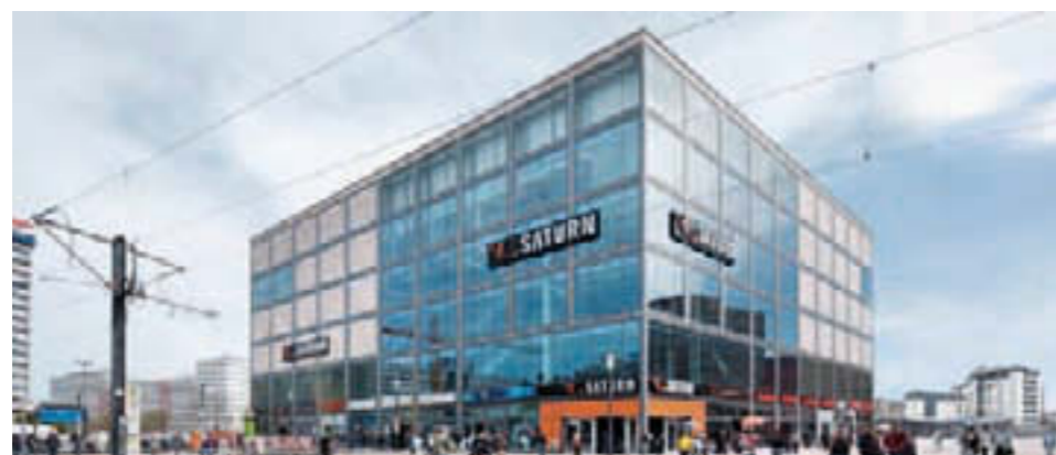
The retail building Die Mitte is located in the heart of Berlin, directly on Alexanderplatz, housing the largest German branch of the Saturn electronic goods store, among other tenants.
